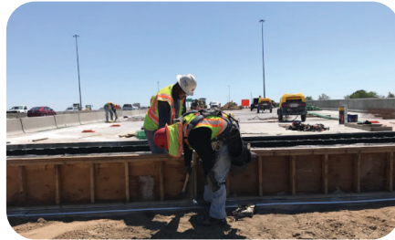
Image 12. Preparation and Pavement of the I-270 Flyover Bridge
