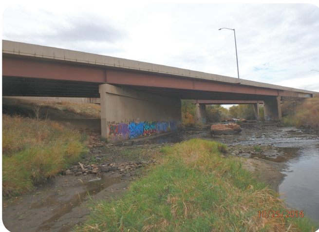
Image 3. I-76 over Clear Creek in Adams County (E-16-LT/LU)
