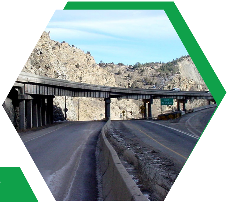
Image 14. Existing I-70 WB over Clear Creek and US 6 in Clear Creek County (F-15-BL)
